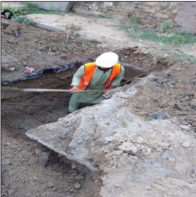
Picture 57: Excavation for laying HDPE pipe
