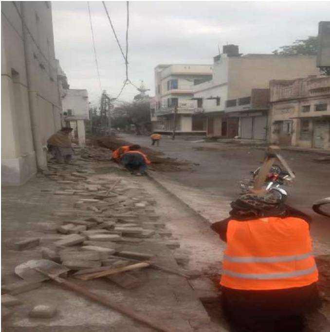
Picture 11: : Road Restoration
