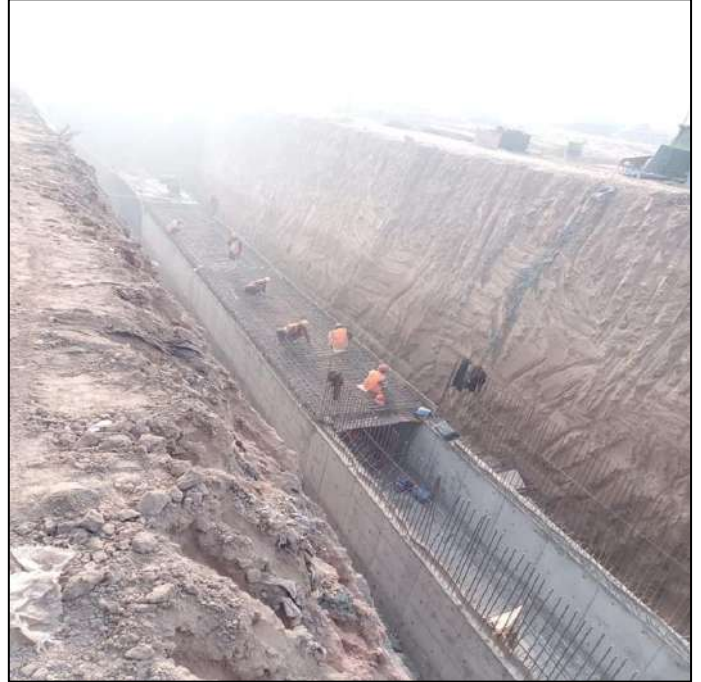
Picture 28: Steel Fixing of conduit top slab
