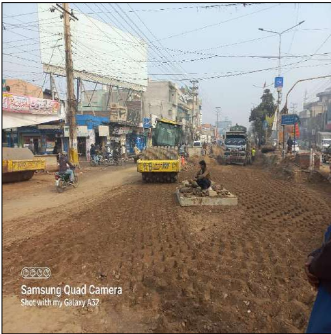
Picture 45: Backfilling of Kotli Behram Chowk @ Kashmir Road
