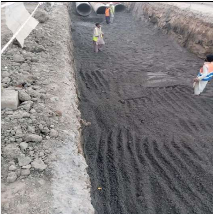
Picture 53: Sand filling under forcemain
