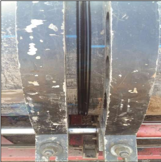
Picture 55: 1200mm HDPE Force Mainpipe jointing
