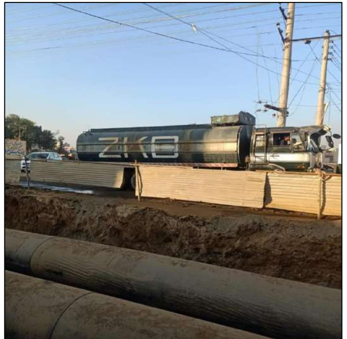
Picture 58: Excavation for Making Gate valve Chamber on Defence Road
