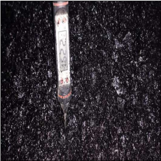
Picture 39: Road Restoration in Progress
