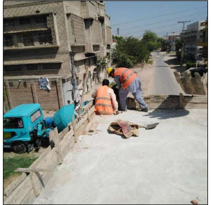
Picture 20: Shuttering of Parapet wall
