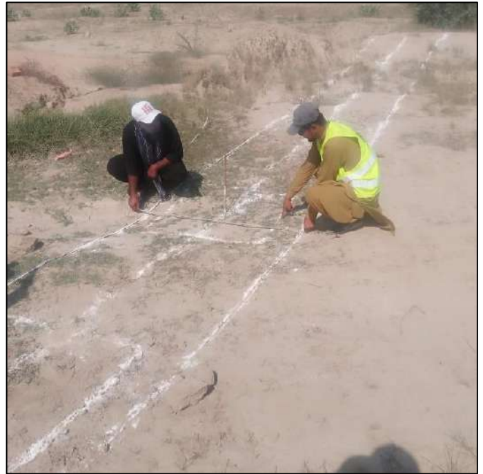
Picture 34: Checking Layout of Boundary Wall of Disposal Station
