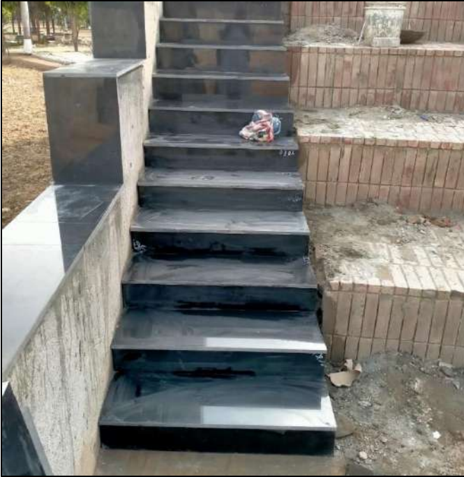
Picture 9: Granite Fixing on stairs of Amphitheatre
