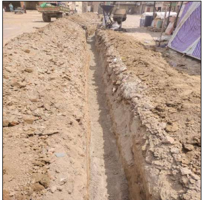
Picture 18: Trench Excavation
