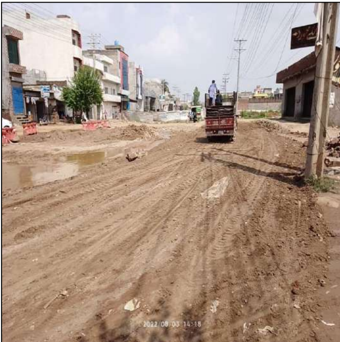
Picture 49: Airport Road
