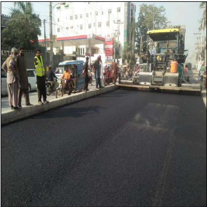
Picture 41: Road Restoration in Progress
