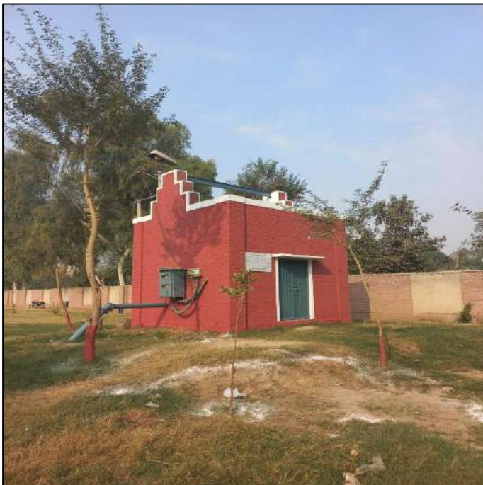
Picture 21: Rehabilitated Tube Well Room
