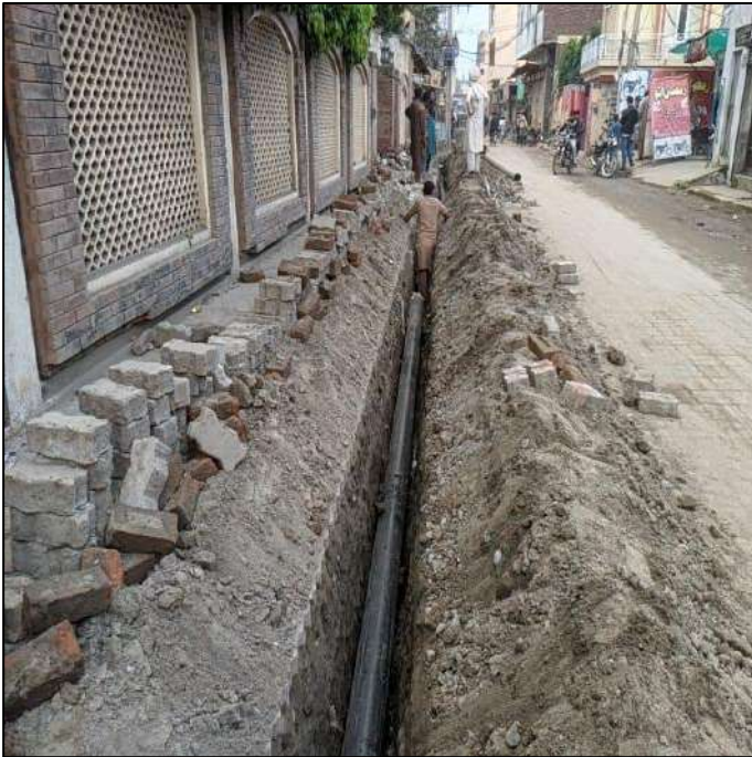
Picture 59: HDPE Pipe laying in UC Miana Pura
