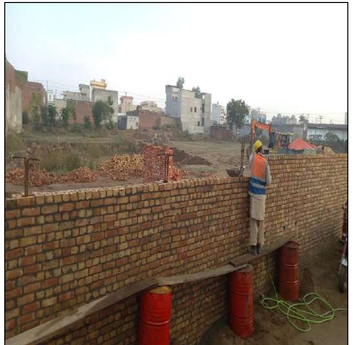
Picture 54: Boundary Wall of Pumping Station
