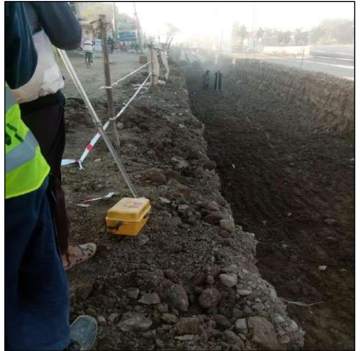
Picture 56: Bed level checking for forcemain
