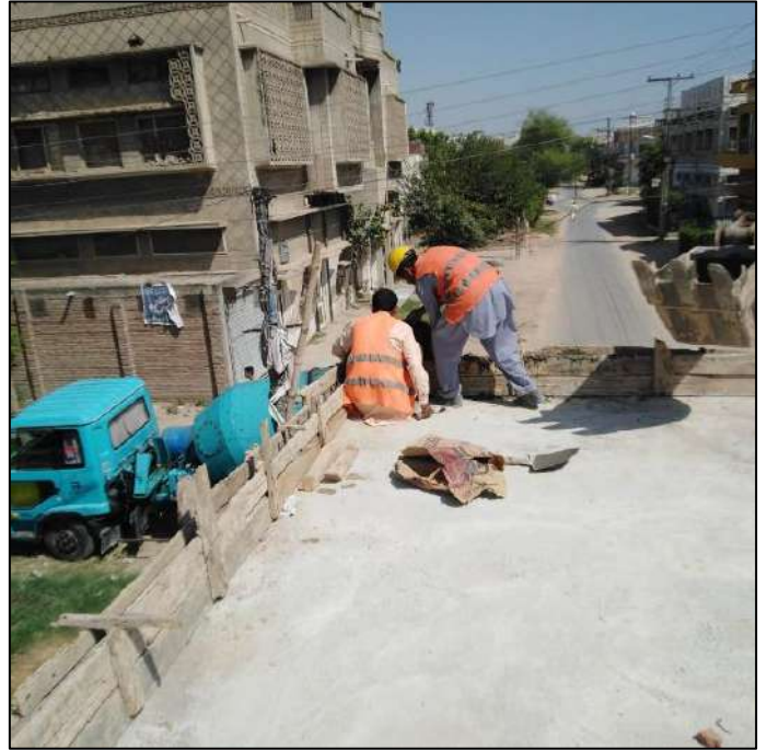
Picture 16: Shuttering of Parapet wall
