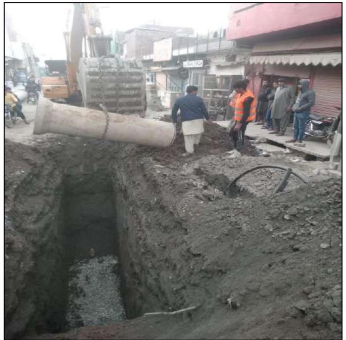
Picture 42: Sewer Laying in Progress
