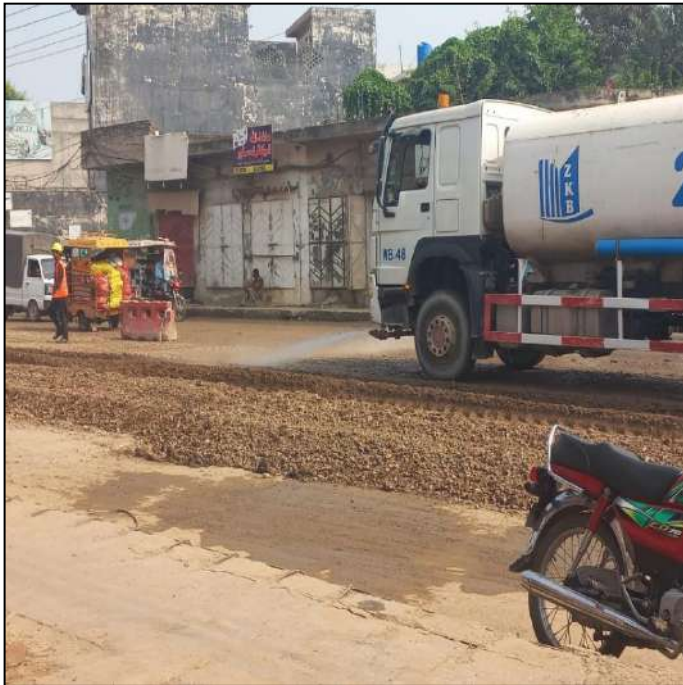
Picture 37: Spreading and Grading of Aggregate Base Course
