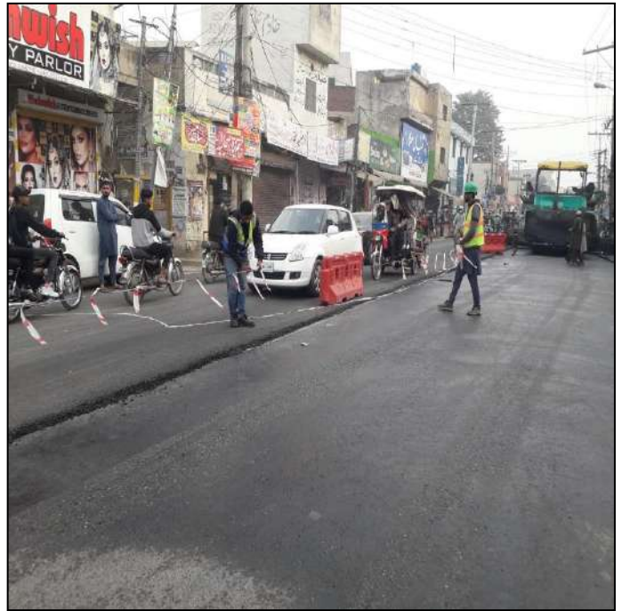
Picture 40: Road Restoration in Progress
