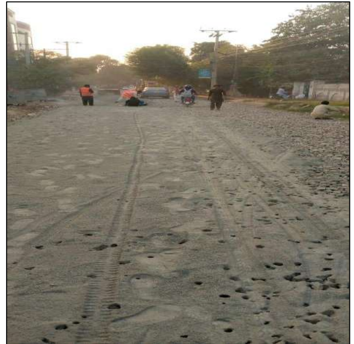
Picture 38: Spreading of stone Dust
