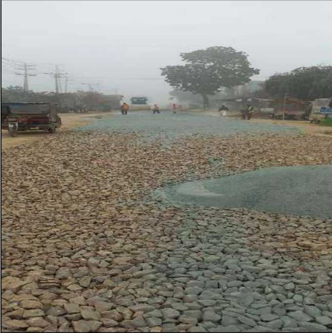
Picture 27: Work of WBM at 54" dia L-2 (KPNS Road) in progress
