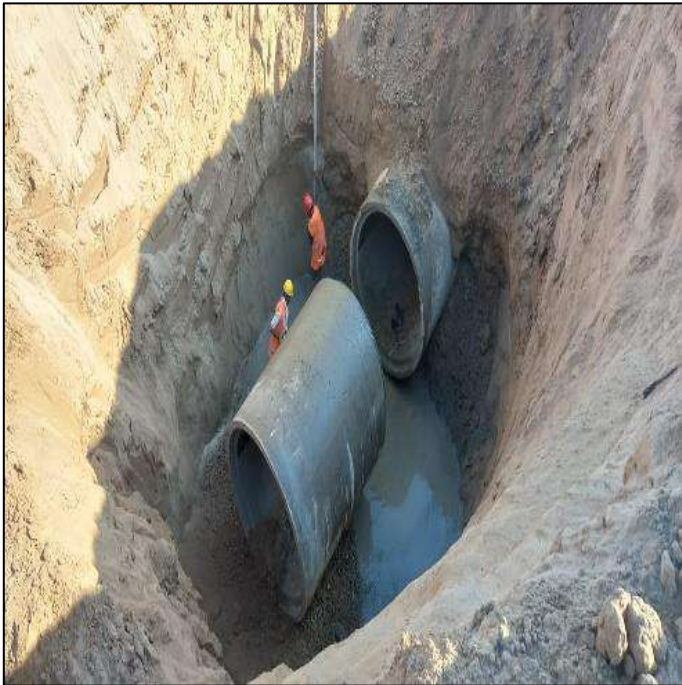
Picture 25: Construction of manhole at 72" dia line
