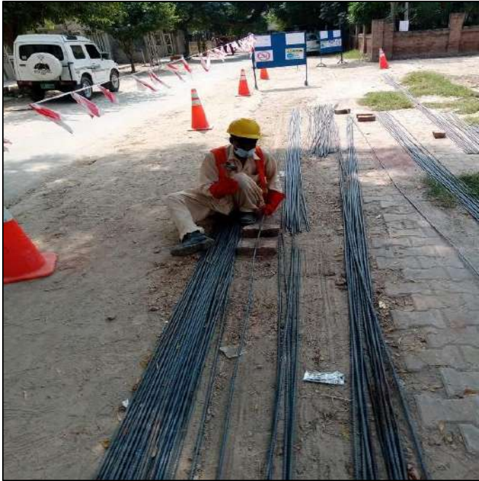
Picture 19: Steel Cutting of staff quarter for Roof
