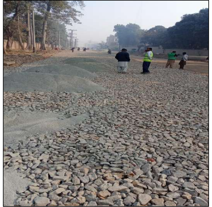
Picture 36: Spreading of the Stone Dust on base stone
