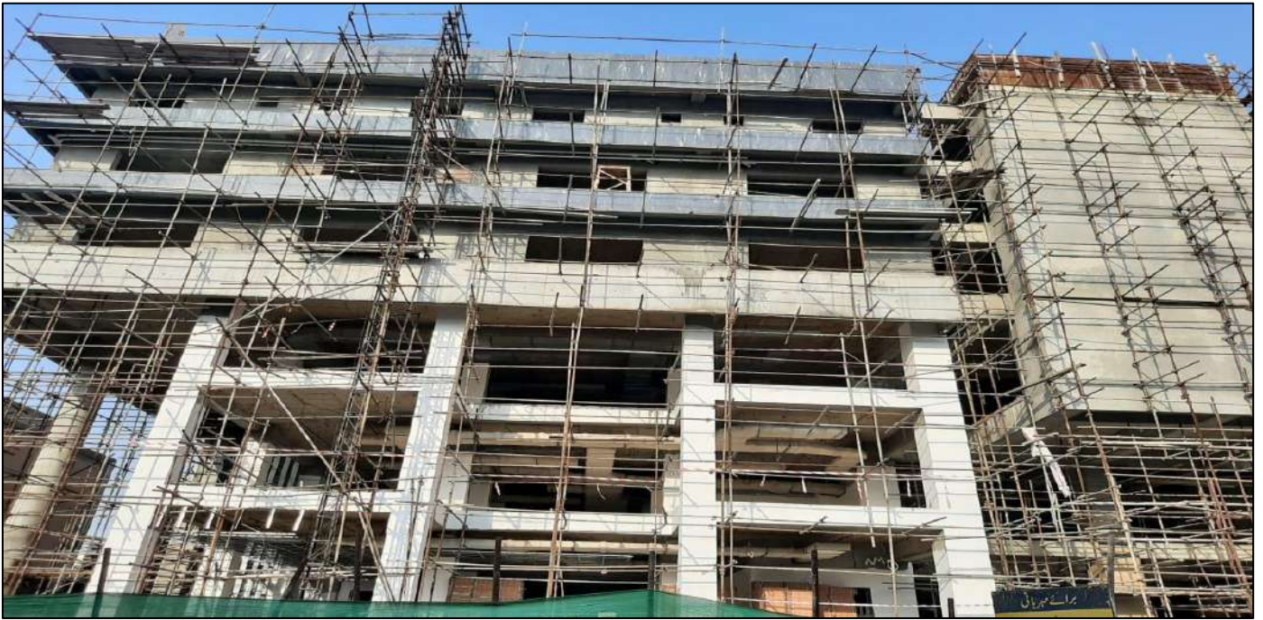
Picture 61: Cladding work on outer walls
