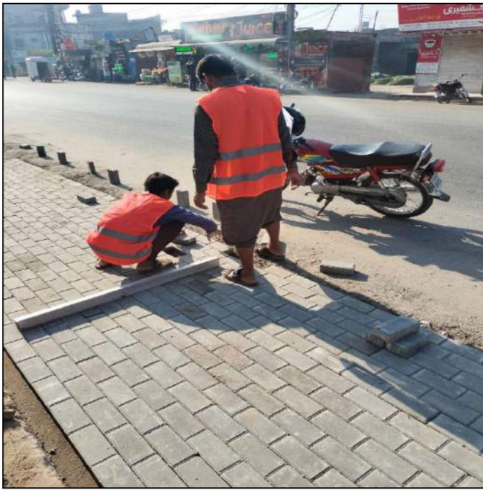
Picture 43: Restored Road
