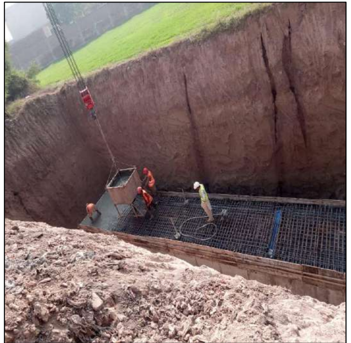
Picture 30: Concrete Pouring for roof slab
