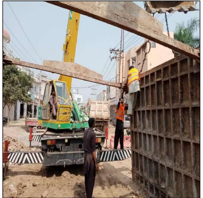
Picture 52: Assembling of Safety Frame for Manhole Excavation
