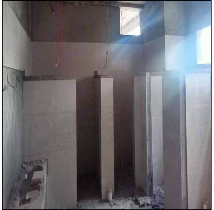
Picture 65: Porcelain Tile work in washroom
