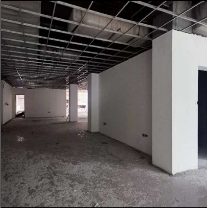
Picture 64: Paint work on walls of Ground floor
