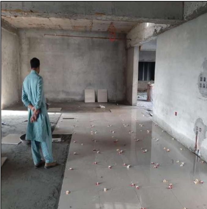
Picture 62: Plumbing work in washrooms at 5th floor
