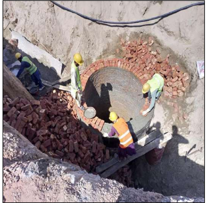
Picture 32: Construction of Manhole at 72' dia. pipe line
