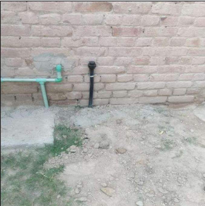
Picture 13: Pump out Test
